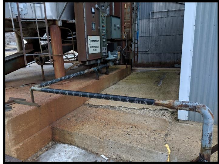
Photo 18 – View of Natural Gas Riser Connected to Grain Drier
