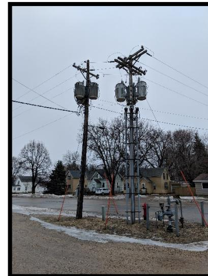
Photo 12 – View of Pole Mounted Transformer
